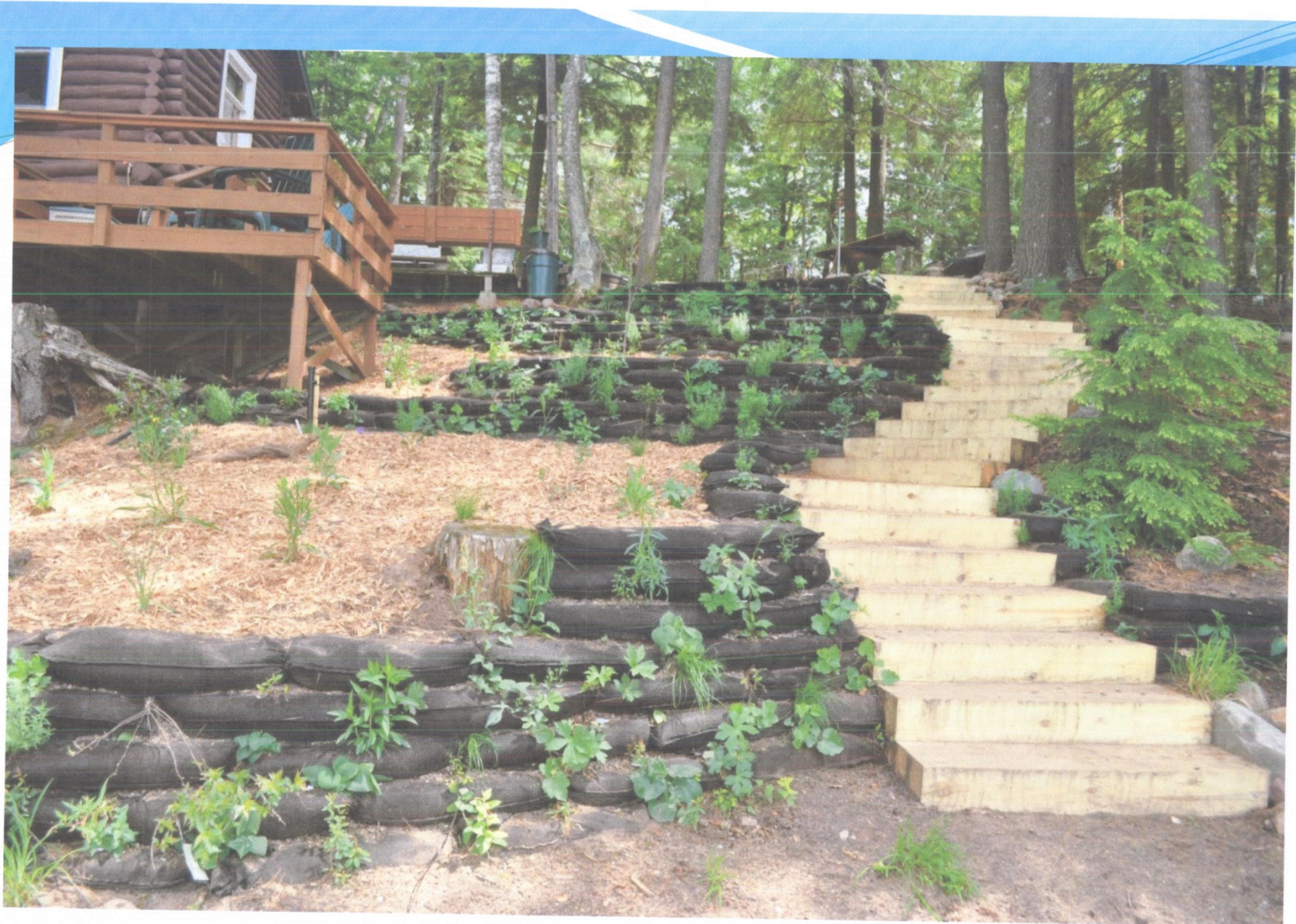
Vegetated Retaining Walls - Geotextile Bags (Install)
