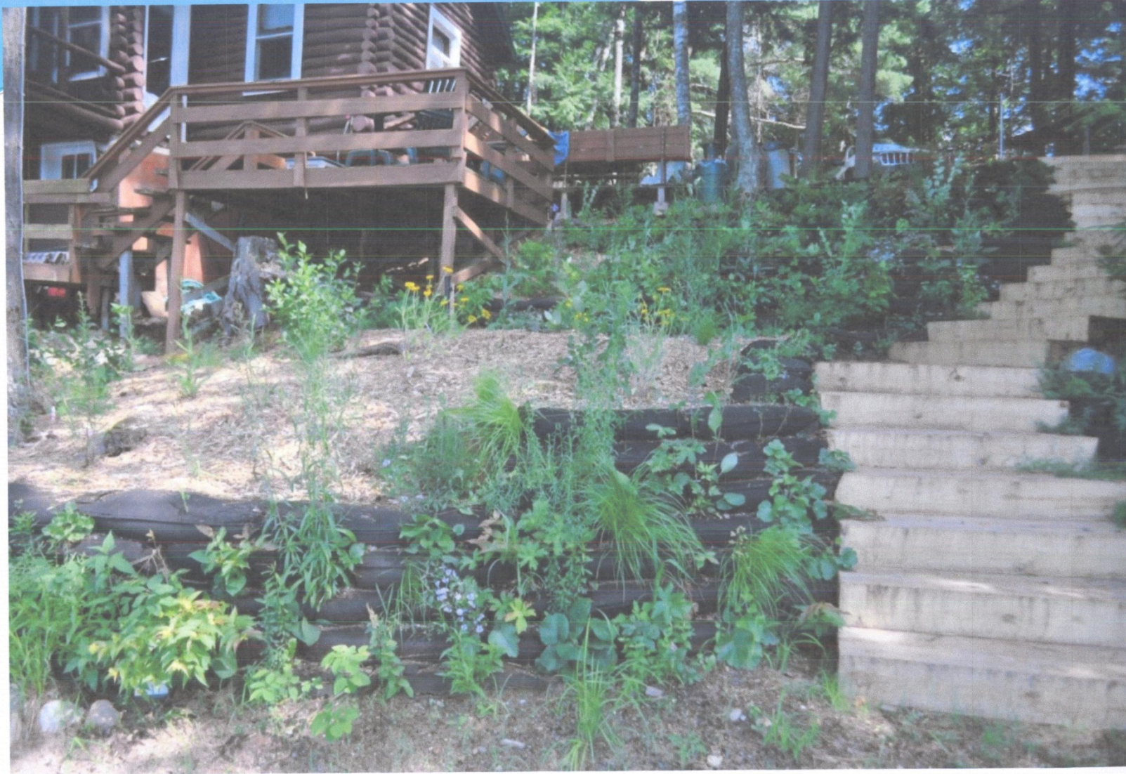
Vegetated Retaining Walls - Geotextile Bags (After)
