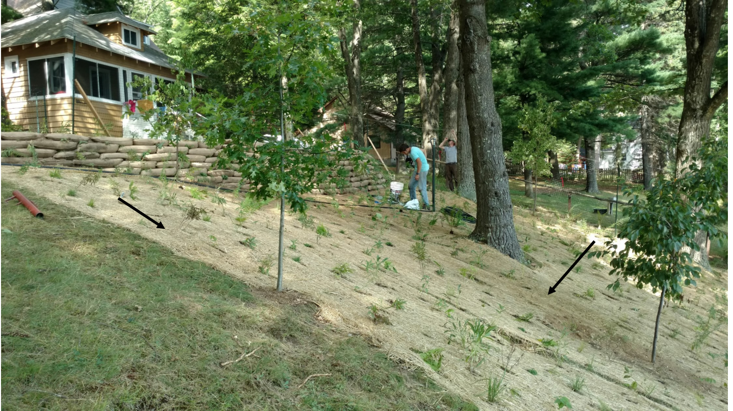
Erosion control blanket in use on a cost share project.
