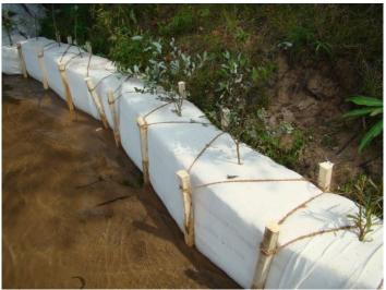
Pounding in the wooden stakes is not the easiest job either. As you can see, we have a hard sand substrate that resists the stakes after about 6" deep. The design specs calls for them, but you may want to consider cables and duckbills. Not sure how tight you can do that though without harming the integrity of the curlex. May be worth a try on a
