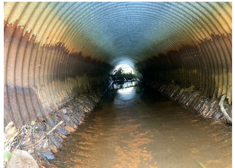
Condition of 4 ft diameter culvert
