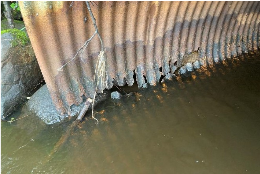
Condition of 4 ft diameter culvert
